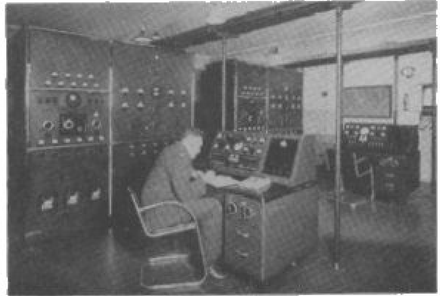
Fig. 9. East Coast CH transmitter room
